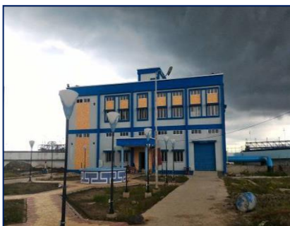
Filter Annex Building
