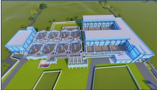
69 MLD Water Treatment Plant
